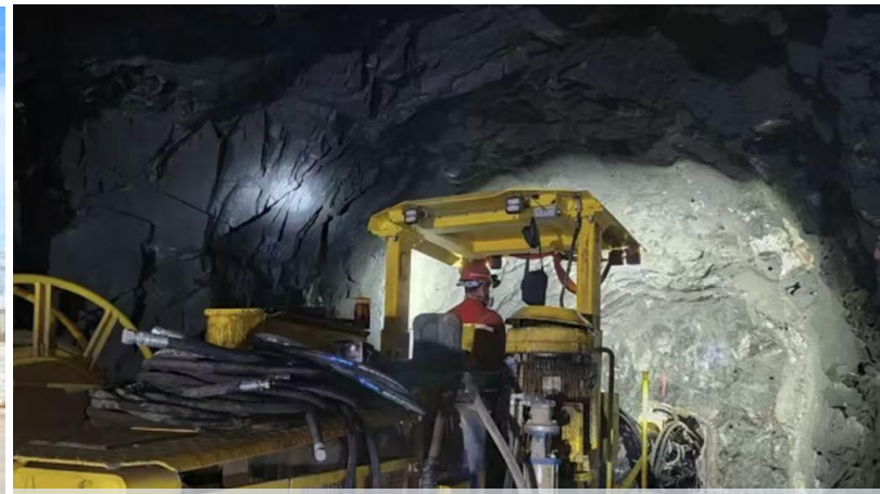
Kuanping Underground Development Underway
