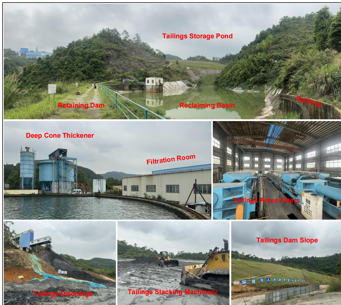
Figure 18.2: Photos of Tailings Storage Facility
