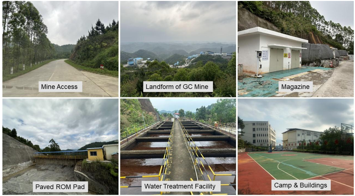
Figure 18.1: Part of Facilities of GC Project
