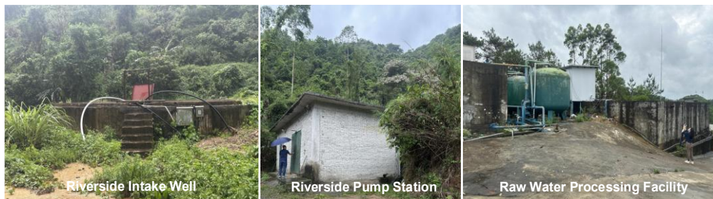
Figure 17.4: New Water Intake, Pumping and Purification Processing Facilities
