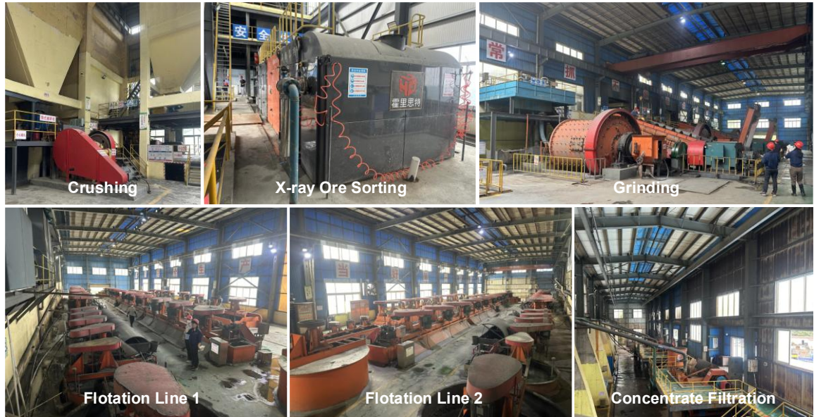
Figure 17.3: Main Production Facility Photos of GC Processing Plant
