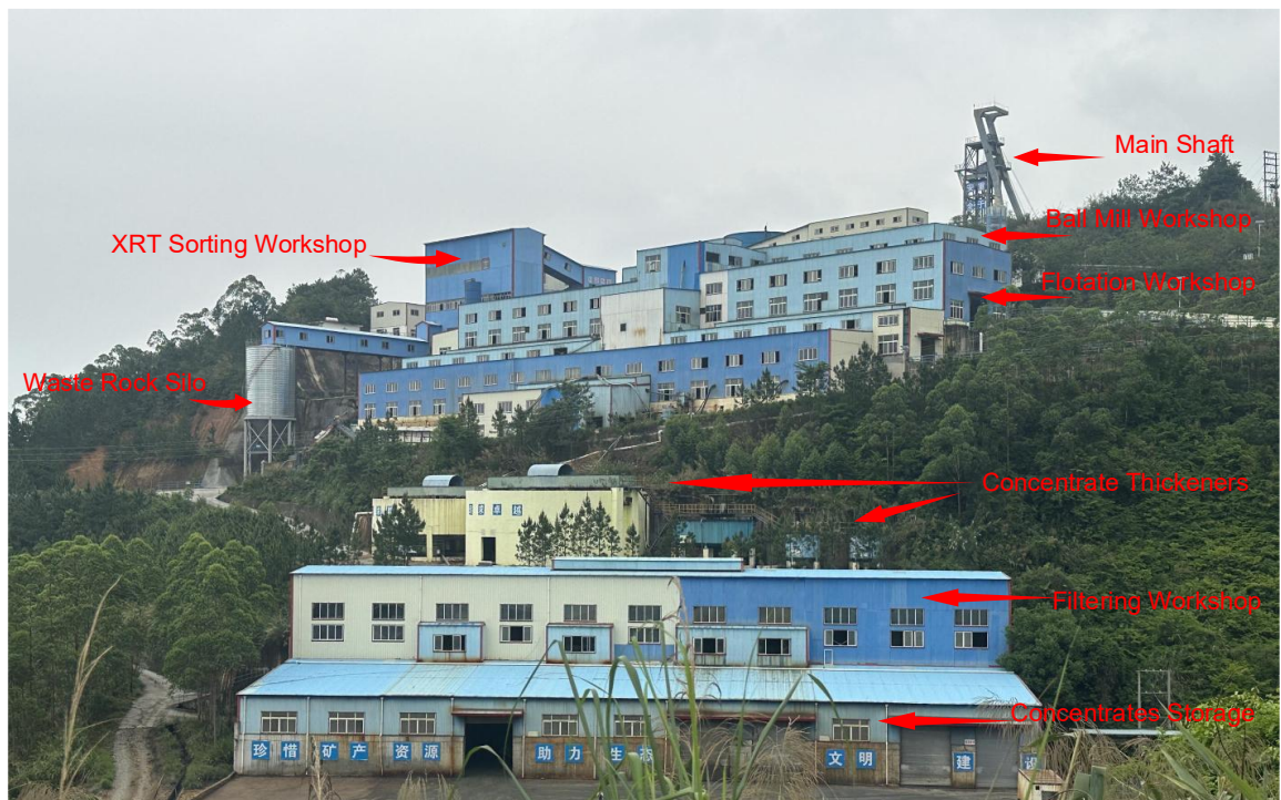
Figure 17.1: Photo of GC Processing Plant
