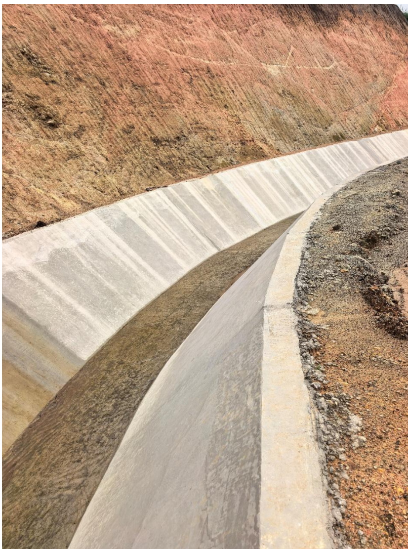
Figure 18.10: As-Built Containment Structures Downstream of the TSF
