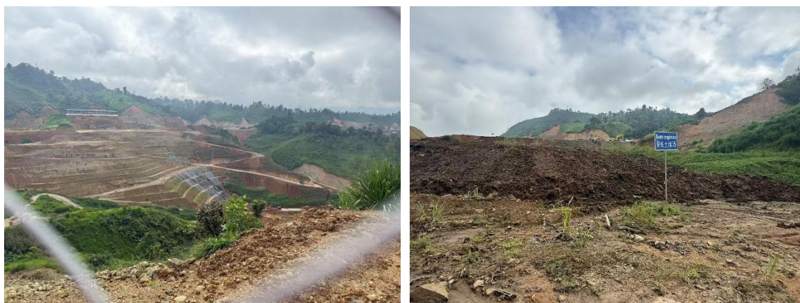
Figure 12.1: Industrial Site Grading
