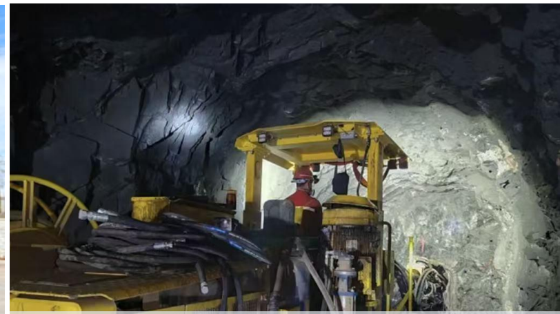
Kuanping Underground Development Underway
